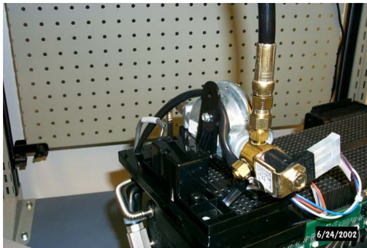
Figure 13: Connecting the Hydrogen Supply
